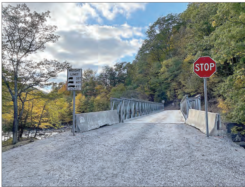
Laneville Bridge over Red Creek attached. USDA Forest Service photo
