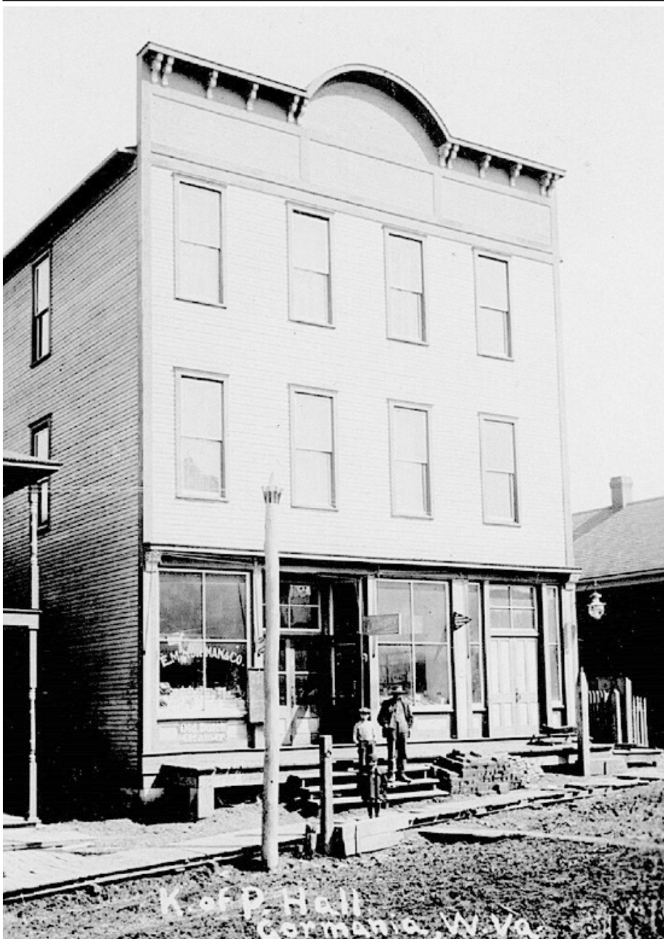
This is the Knights of Pythias Hall at Gorman, WV. On the first floor is a business E. M. & Co. Below a window is an advertisement for Old Dutch Cleanser. A sign by the door reads Laundry. Notice that the streets are not paved and there is a boardwalk. The tall pole in the center of the photo is an electric pole. At least four insulators are on the top of the pole and there are at least two wires connected to the pole. Ideas, comments, suggestions, or items to share contact Tim Turner at (304) 478-3389.
