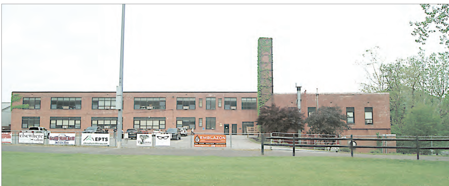
Woodlands Development and Lending has proposed a development plan for the School Board building that would turn a portion of the structure into 15 apartment units for residents making less than 60% of the area's median income.
