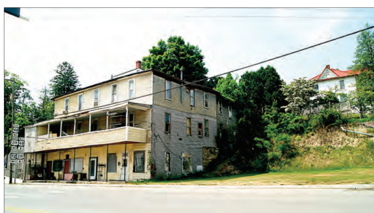
The City of Parsons just authorized the demolition of three properties within the city. The building at 193 Main St is one of three slated for demolition.
