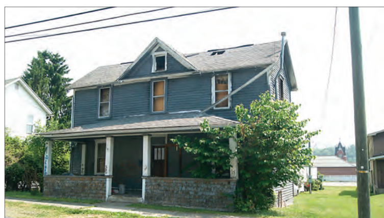
The Parsons City Council voted on Tuesday, June 6th to demolish three properties within the city. The property at 170 Spruce Street was one of three slated for demolition by the city.
