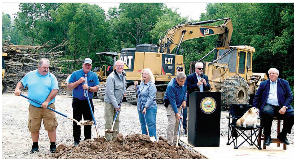
Tucker County Commissioners Fred Davis, Tim Knotts and Mike Rosenau greet Governor Jim Justice and Baby Dog following the groundbreaking for the new section of Corridor H in Tucker County.
