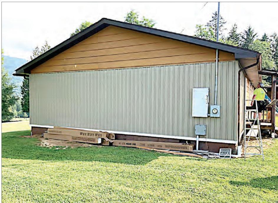
New siding is going up on the boy's dorm at Camp Kidd.
