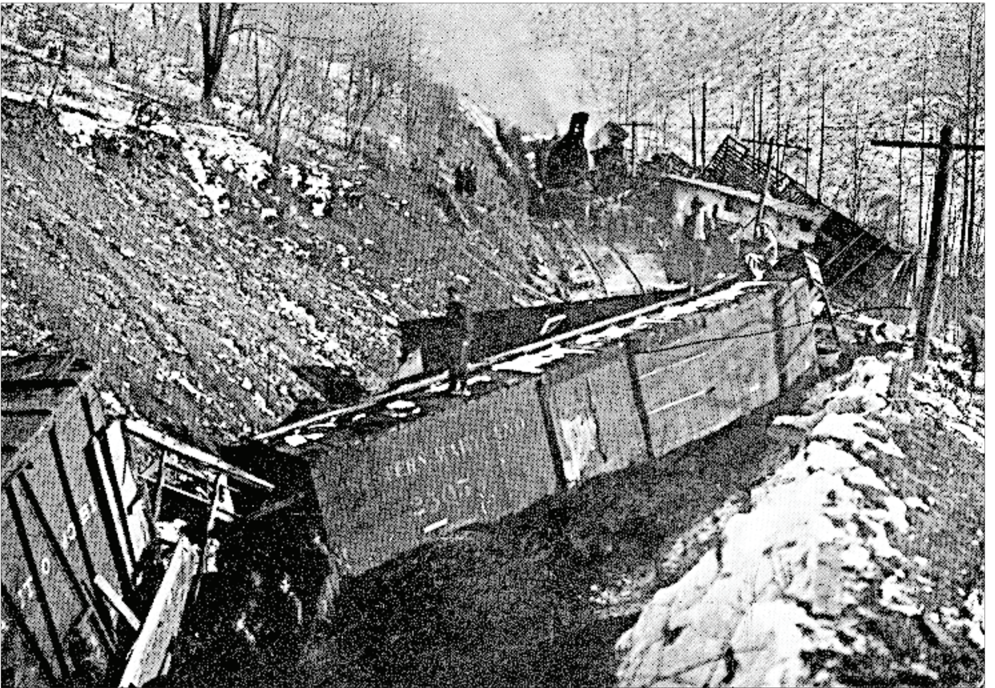
This is a postcard dated May 19, 1919. The tail end of wreck on the mountains 4 miles east of Hendricks. Wreck train in the rear clearing track. This train ran three miles before leaving the rail and was making 70 miles per hour. The brakeman was killed, he was under the wreck two days. Ideas, comments, suggestions, items to share contact Tim Turner (304) 478-3389.
