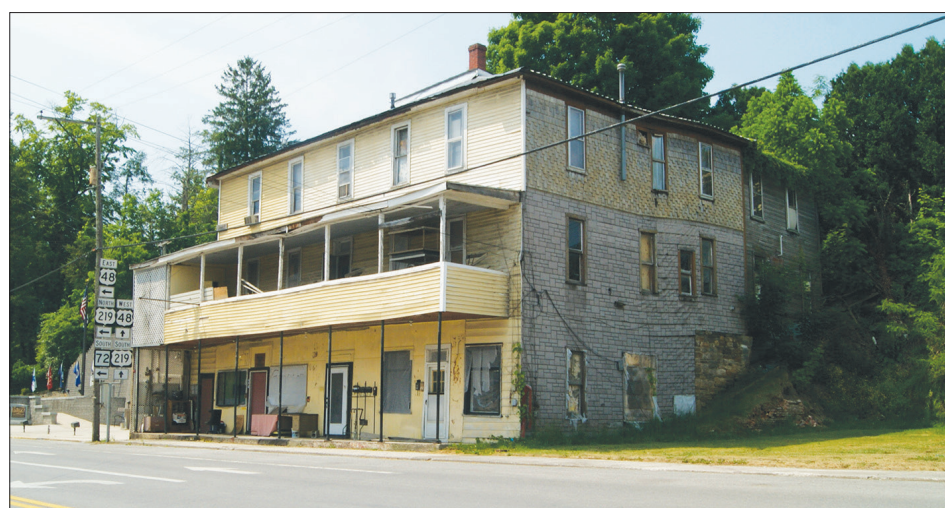
The building at 193 Main St., pictured, will soon have demolition barriers placed around it as initial demolition work begins. Smokey Joe Enterprises, LLC of Beverly was one of two companies contracted by the city to demolish three derelict buildings in Parsons. The Main St. building will be the first to begin coming down from the civic improvement initiative.
