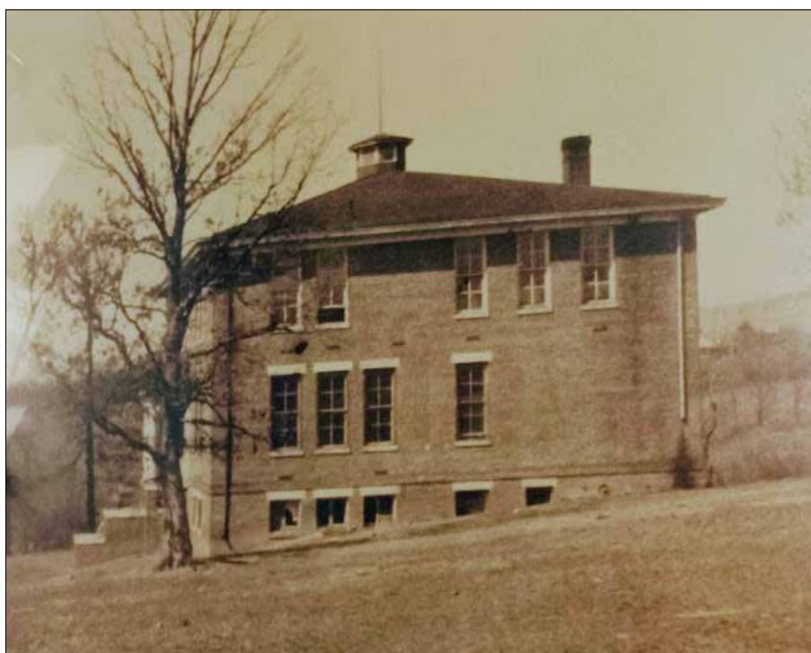
Side View of Square School on Chestnut Street.
