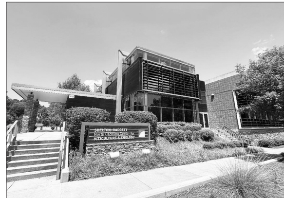
The Shelton-Badgett North Carolina Center Viticulture & Enology located at Surry Community College is a state-of-the-art building with a climate-controlled wine cellar, microbiology labs, assembly hall, and a 2,500-gallon licensed and bonded teaching winery. If you’d like to find out more about the Viticulture and Enology program at Surry Community College, visit surry.edu/wine or call (336) 386-3391.
