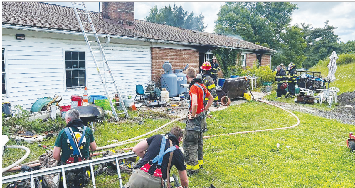
Damage from the blaze was contained to half of the brick ranch-style house.
