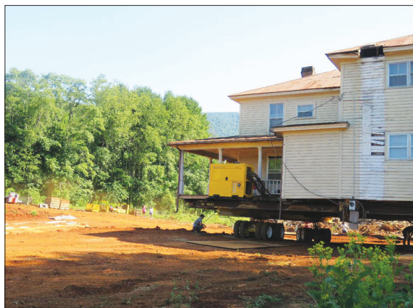
The house with the wheels to move it in place. (Photos by Joanne Hill)
