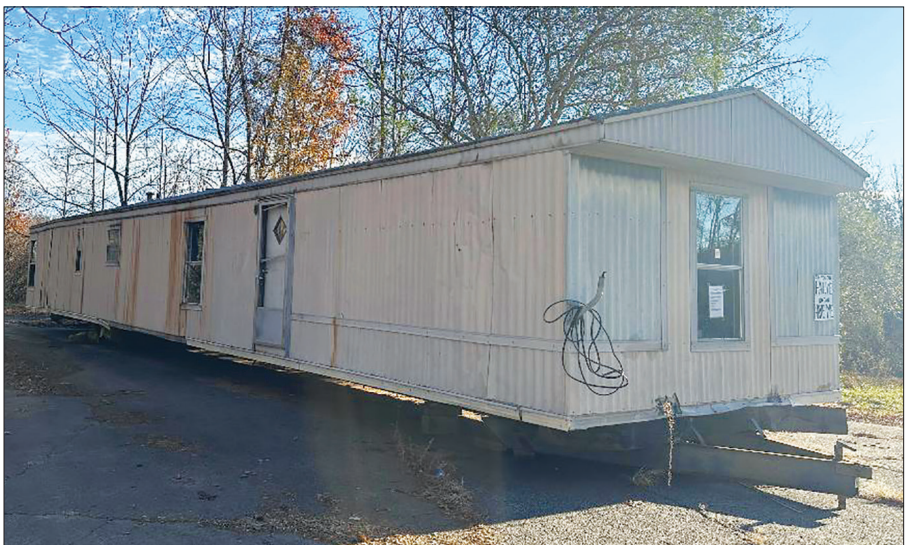
A mobile home has been parked near the Virginia 8/103 intersection for months. (Contributed photos)
