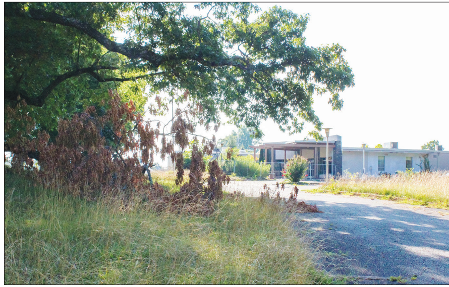
The hospital property appears unkempt and unmaintained.
