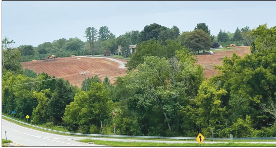
A solar facility is being built on the former Bassett Country Club property. (By Ray Reynolds)
