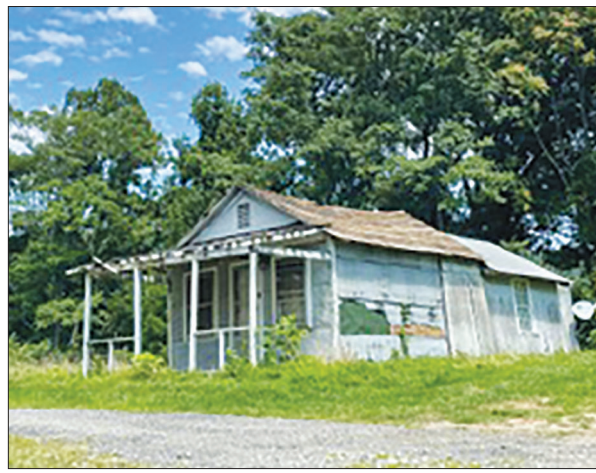
The humble abode known to many local residents as Blind Man Martin house is pictured before it was demolished to the last splinter as work on the U.S. 58 project continued its march.
