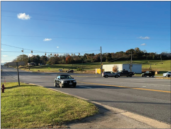
Overhead flashing beacons were added to the intersection of U.S. 58/Virginia 680 in 2017. The beacons were designed to enhance visibility.
