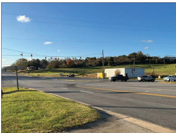
Overhead flashing beacons were added to the intersection of U.S. 58/Virginia 680 in 2017. The beacons were designed to enhance visibility.
