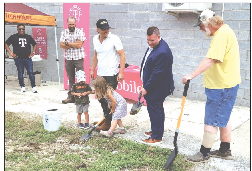
COURTESY PHOTO The groundbreaking for the Craig County Farmers Market has many Craig residents excited. From left: A T-Mobile representative Mac Hobbs, Craig County Supervisor Jason Matyas, farmer Ty Walker, Economic Development Authority chairman Jordan Labiosa and New Castle Town Councilman Ed Lee. The two children are Gratton Walker, age 3, and Eve Walker, age 5.
