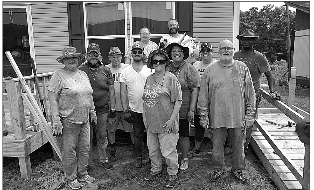
PICTURED IN FRONT of Patti Keatley's home are some of the good-hearted members from Mill Church of the Nazarene in Noblesville, Indiana. The mission team came to Marlinton to help build ramps and make small home repairs for a few of the families here. Team members raise money all year long for the trip – to pay for lodging and some of the materials they use. They give up vacations and time with their families to do this work. Keatley, standing in back with her son, Greg, said, "These people have been so kind and wonderful." L.D. Bennett photo
