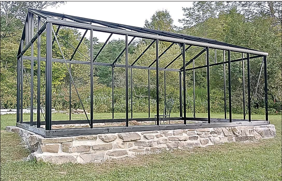
FORMULATING THE PLACEMENT of natural stone to construct a foundation for a greenhouse. M. Phillips photo
