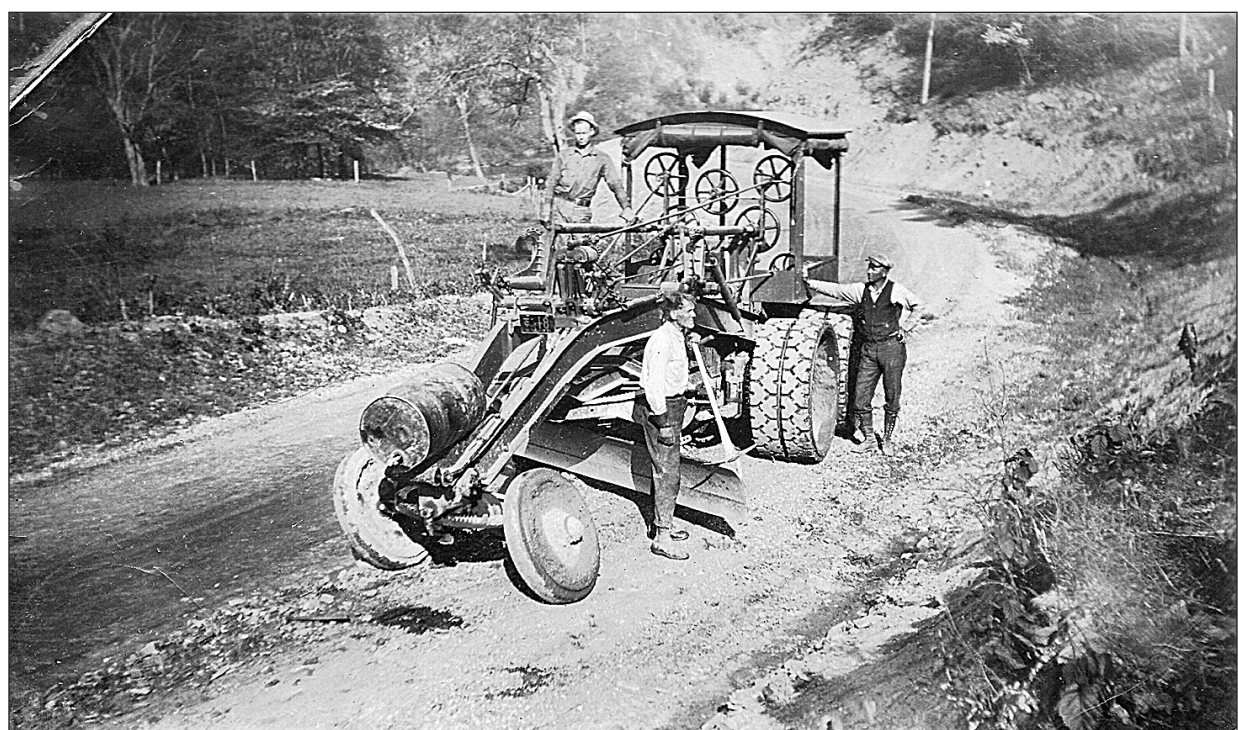
WILLIAM HILL, LON Hubert Kershner and Guy Thomas working road construction near Marlinton, W.Va. (Photo courtesy of Kay Beverage; ID: PHP003809)
