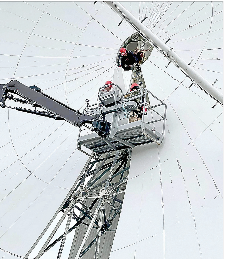
MEMBERS OF THE Green Bank Observatory crew remove panels from the Ny-Ålesund 30-meter telescope as the first part of the deconstruction of the decommissioned instrument. Photos courtesy of GBO
