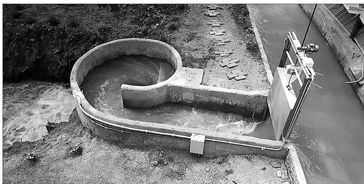
THE COMPANY THAT developed the Vortex Turbine states, “A single turbine can generate from 15 to 70 kW of constant energy around the clock.” This innovative design only needs a low flow and low head and has minimal impact on the environment. Photo courtesy of pinterest
