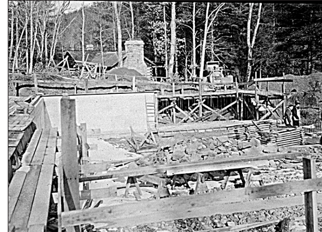
Photos courtesy of Preserving Pocahontas The Watoga swimming pool under construction by the Civilian Conservation Corps. At right, the pool and bathhouse was the last major project of the CCC at Watoga. This photo was taken in 1948.
