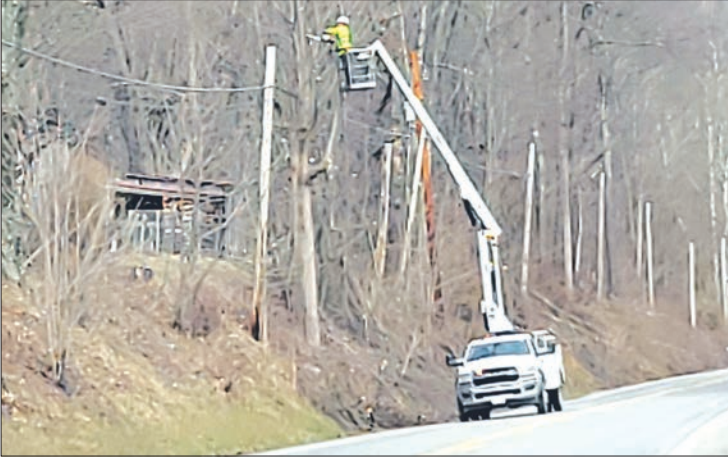
One of the issues addressed in Pendleton County's formal complaint to the Public Service Commission against Frontier Communications was failure to maintain their lines free of brush and tree limbs. Frontier appears to be taking the requested remediation seriously. Last Wednesday, a contractor for Frontier was hard at work clearing branches from Frontier's line alongside Route 33. The previous week, falling tree limbs had dislodged a line from the poles and left it hanging about eight feet above the roadway, closing one lane to traffic for several hours. This is currently the only line which carries Pendleton County's emergency 911 communications, although Pendleton County's complaint asks for a second line to be built on a separate route, to provide redundant back-up in the event that this line becomes disabled, as has happened multiple times in the past when accidents involving runaway trucks on Allegheny Mountain have taken broken utility poles and severed the cable.
