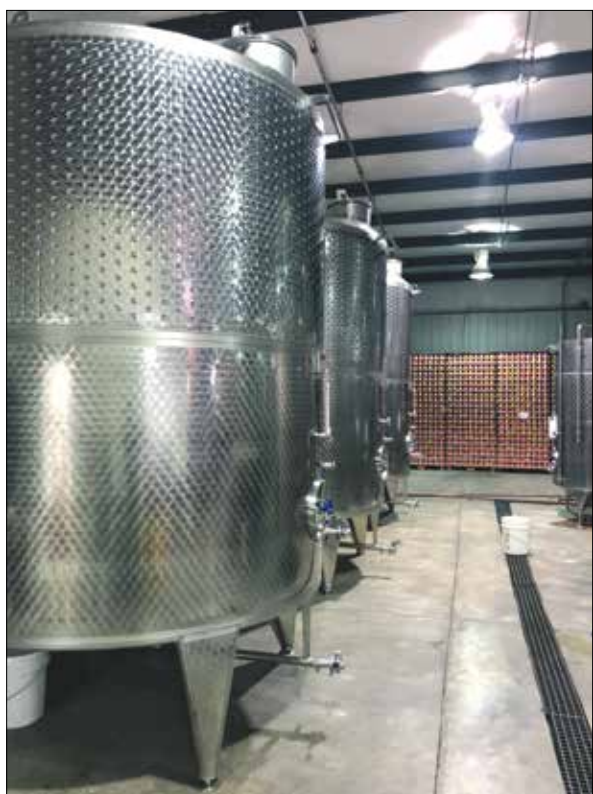
New 10,000-liter tanks were installed for Swilled Dog's cider production. Photo by Walter Hojka.
