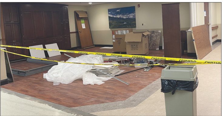
Construction of the new hall at Pendleton Manor is underway.
