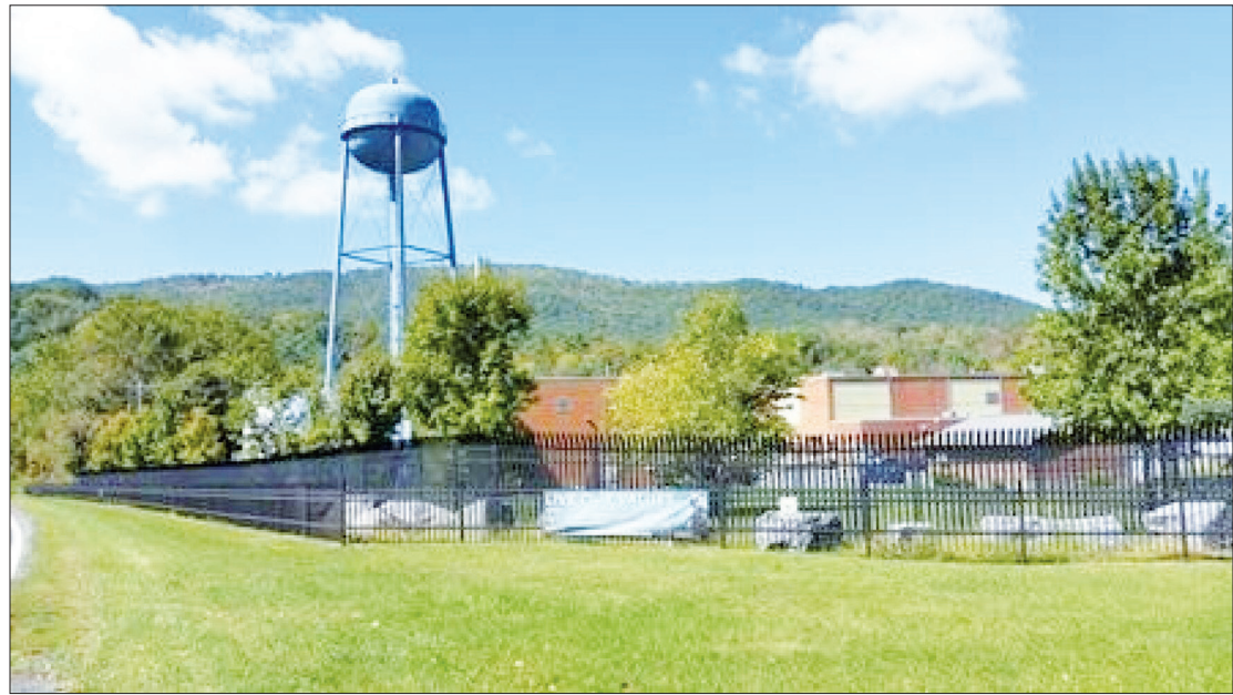
Pendleton County officials remain optimistic that the right tenant will come to the former base at Sugar Grove.
