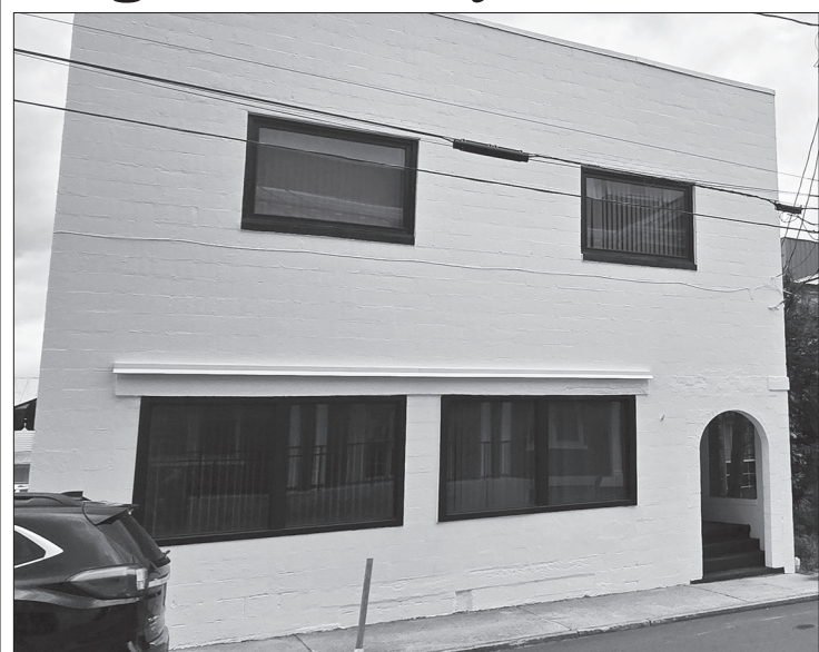
With exterior work completed, the SRRDA will soon see a renovation of the first floor of its Franklin Innovation Hub.
