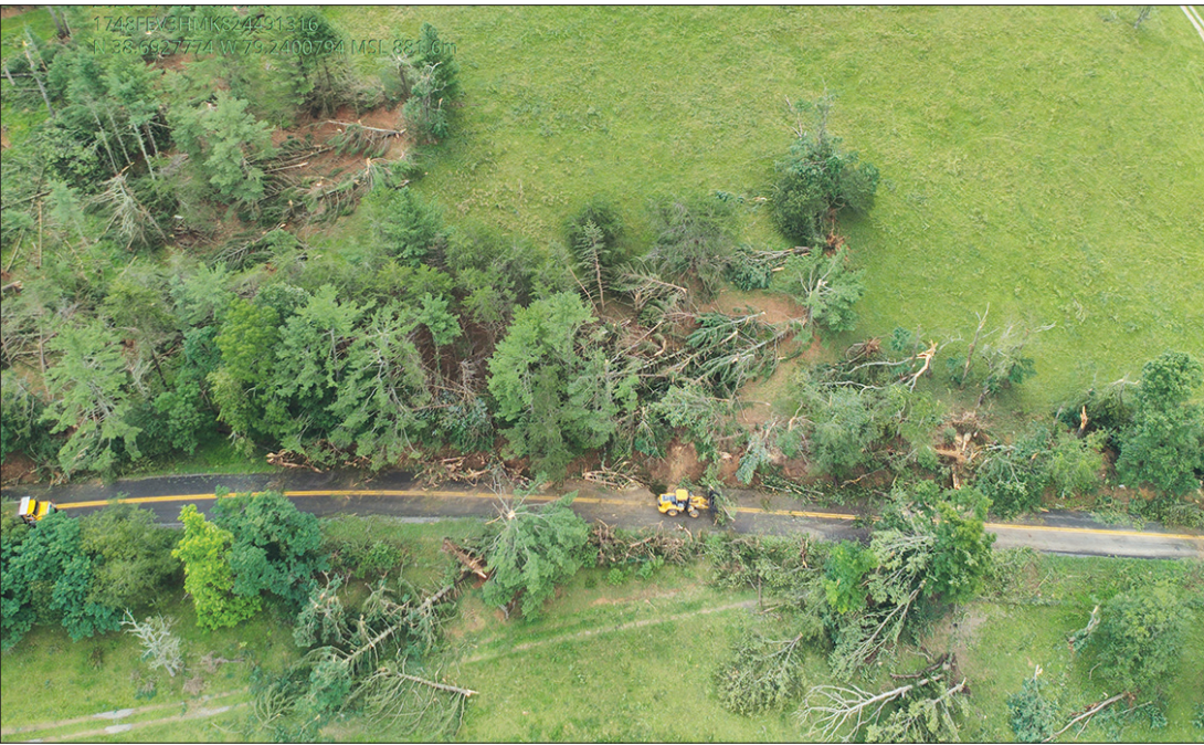
West Virginia Department of Highways' crews work to clear Troublesome Valley Road.
