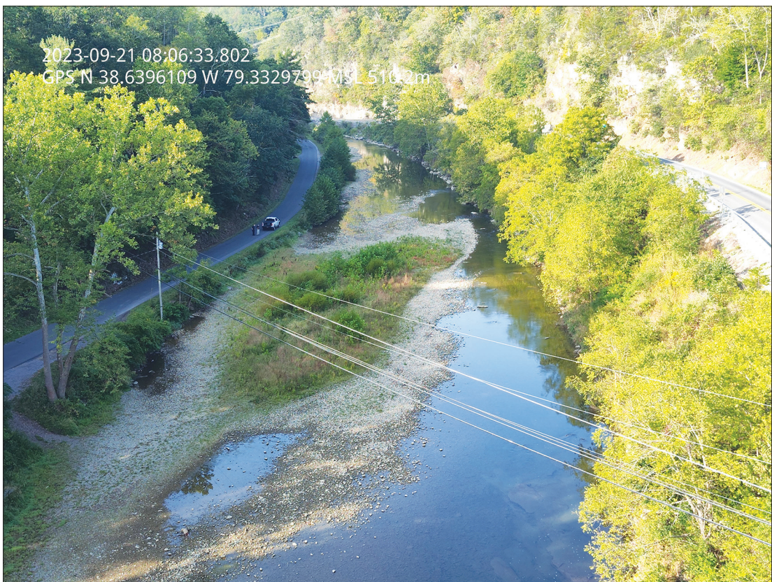
This major obstruction of trees growing just upstream of the low water bridge in Franklin has Pendleton County officials concerned. Those worries have been expressed to federal officials. Photo courtesy of the Pendleton County Office of Emergency Management.
