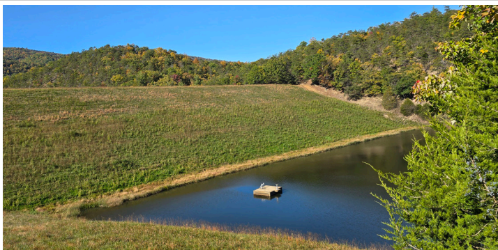
South Fork Dam Site Four near Peru Hollow during heavy storms can hold large amounts of water out of the South Fork River. It and dams like it help to prevent floods and reduce loss of life and damage during disasters.
