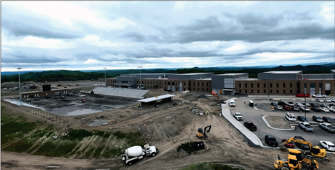
Construction continues in mid-May at Southern Gap High School as large work trucks and crews remain active in front of the building during ongoing site development.
