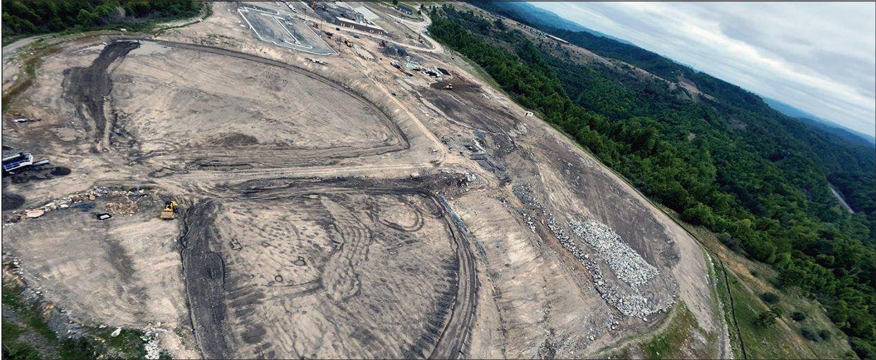
Softball and baseball fields at Southern Gap High School began to take shape in mid-May.
