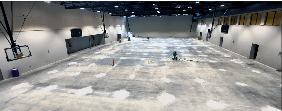
Photos courtesy of CTE students from the BCCTHLC An updated view of the gymnasium shows progress in mid-May at Southern Gap High School, where interior work continues ahead of final finishing touches.
