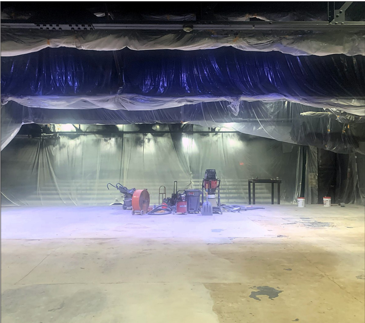
The CAM's stage is shown from backstage, looking toward the audience, on July 1, as renovation work was underway. The theater curtains were pinned up and wrapped in protective plastic while the stage floor had been stripped in preparation for refinishing, part of a series of behind-the-scenes improvements designed to preserve and enhance the facility for future performances.
