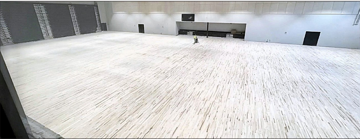
Construction Superintendent Tim Burge shows Buchanan County School Board members the nearly completed gymnasium floor at Southern Gap High School during a July 13 construction update. Crews were preparing to sand, stain and seal the hardwood floor as work enters its final stages before the school's Aug. 21 opening.
