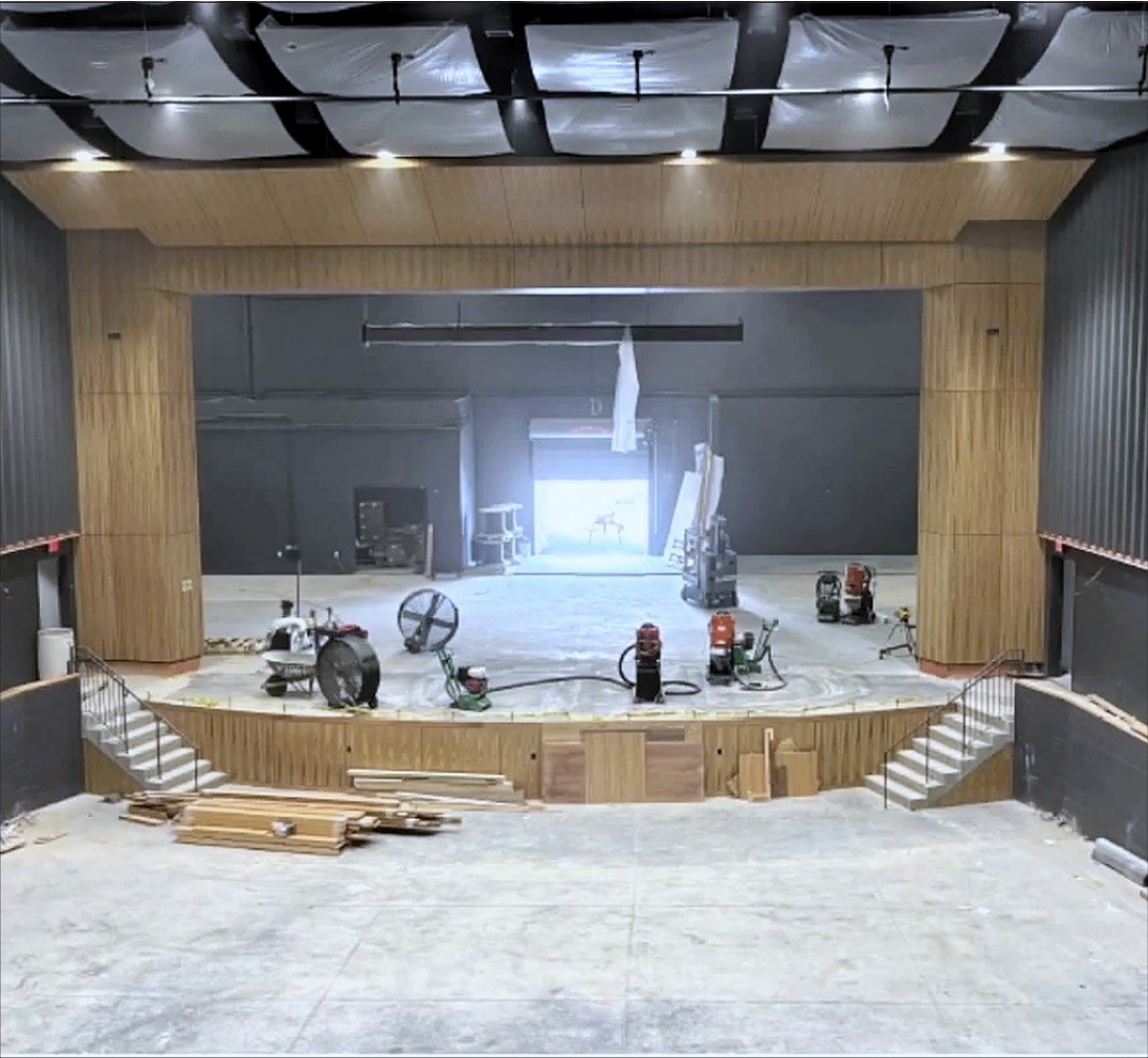
The auditorium at Southern Gap High School is among the many areas nearing completion as crews put the finishing touches on the new campus. Construction Superintendent Tim Burge shared images of the facility with the Buchanan County School Board during a July 13 progress update.
