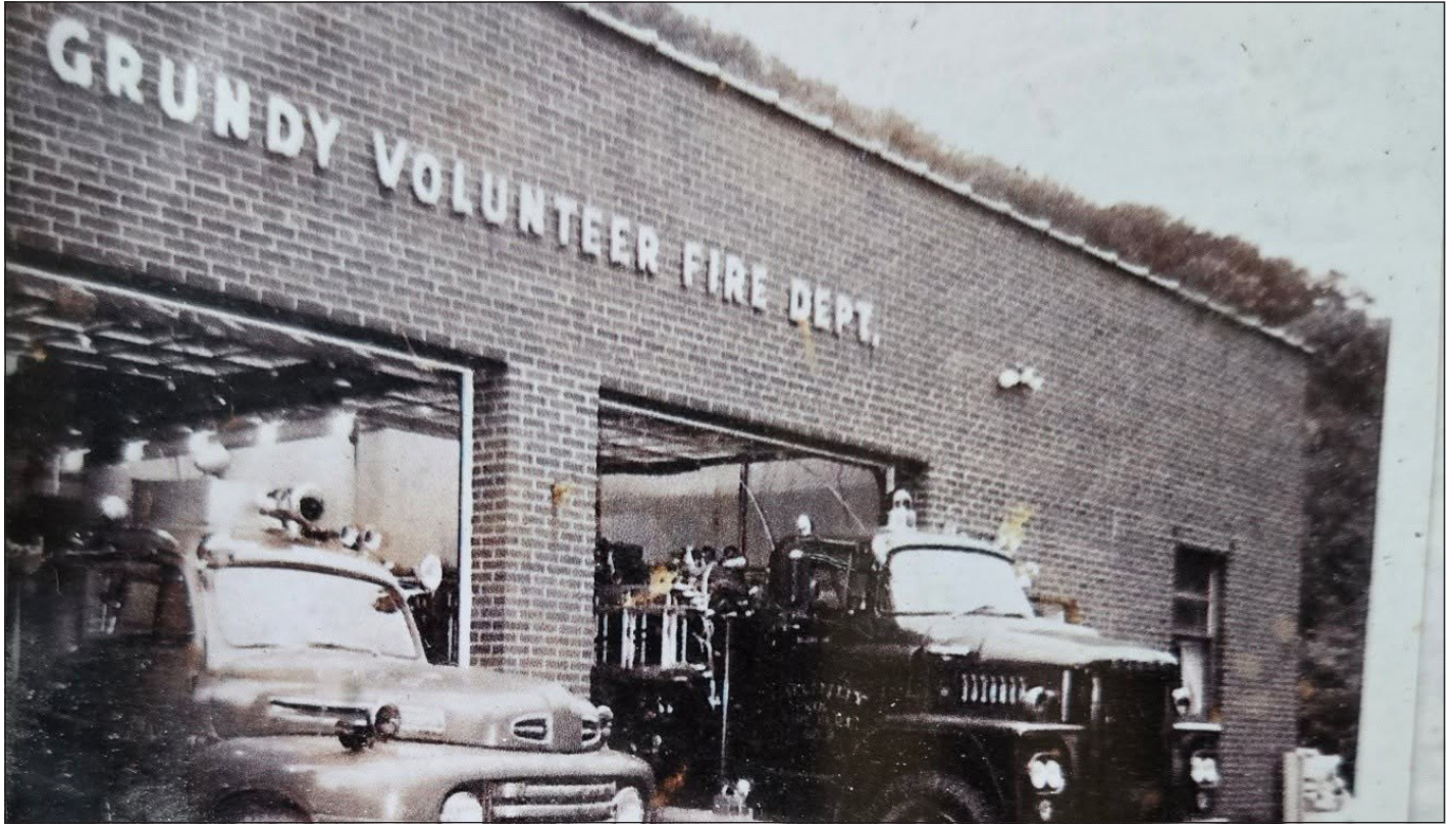
An early photograph of the Grundy Volunteer Fire Department station shows two fire trucks extending from the building's bays. The department was established in 1947 (photo courtesy of GVFD).
