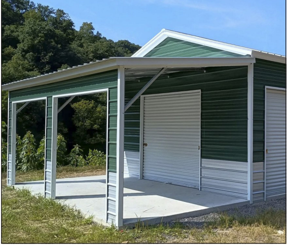
The new Buchanan County Farmers Market is located behind the large Southern Gap sign at the entrance to Southern Gap Road in the Prater District. The 20-by-30-foot building features a 10-foot porch and is expected to open soon (Contributed photo).
