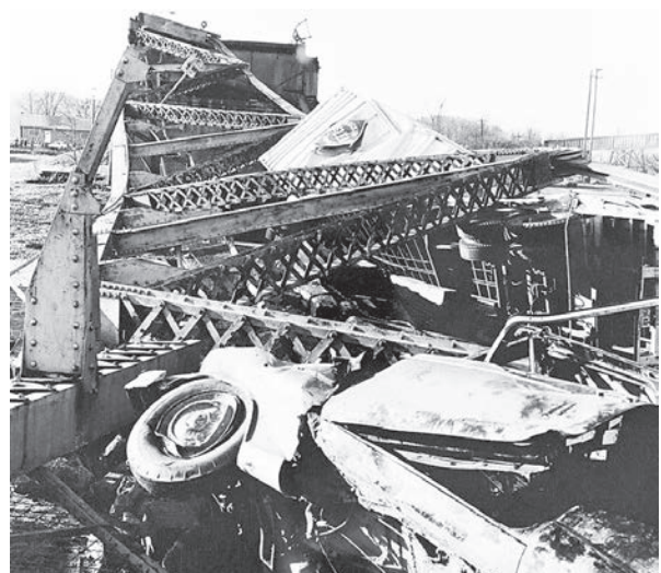
Wreckage of the Silver Bridge at Pt. Pleasant, which collapsed on Dec. 15, 1967, killing 46 people.
