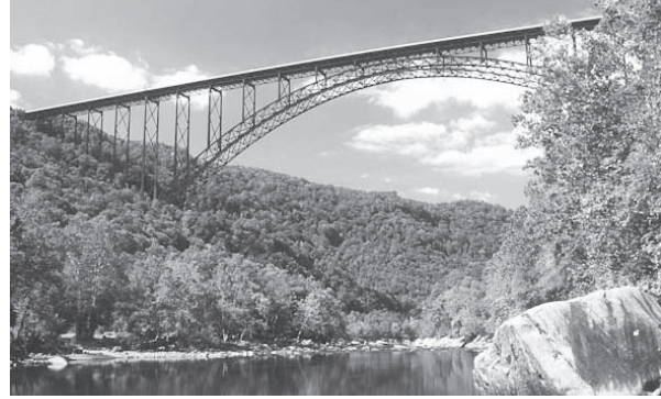
Construction of the New River Gorge Bridge was completed Oct. 22, 1977, after three years of work.
