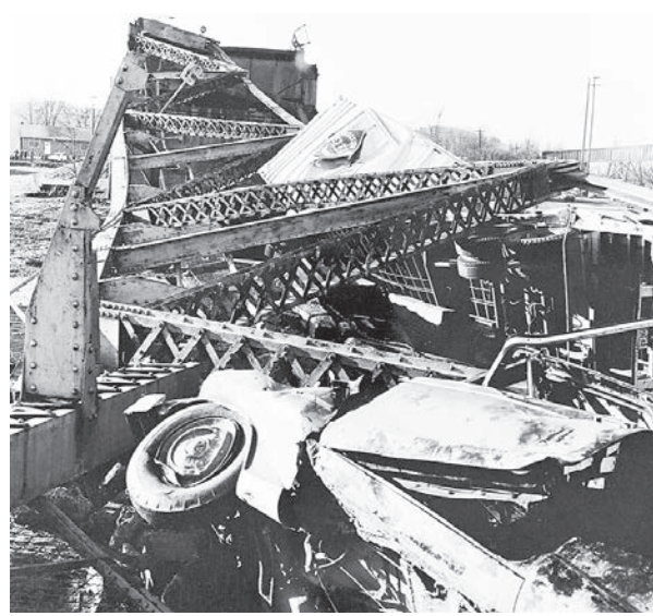
Wreckage of the Silver Bridge at Pt. Pleasant, which collapsed on Dec. 15, 1967, killing 46 people.
