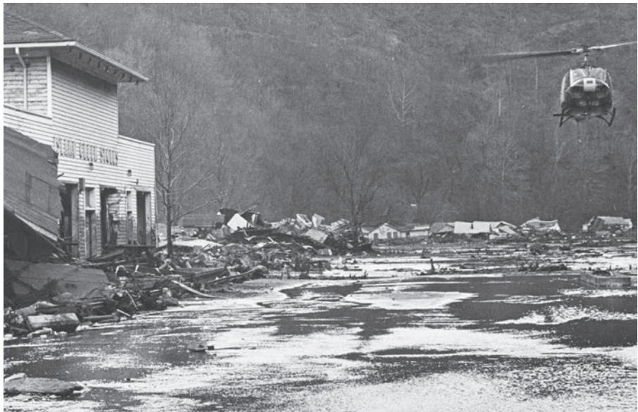
A coal waste dam collapsed on Feb. 26, 1972, sending water, coal refuse and silt into the Buffalo Creek valley, killing 125 people.
