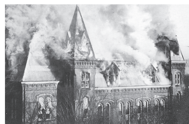
The state capitol building in Charleston was destroyed by fire on Jan. 3, 1921.
