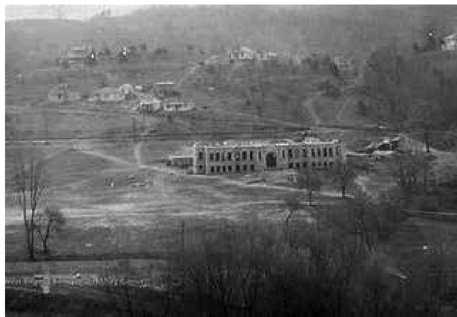
A long-distance picture of construction of the school about 1923.
