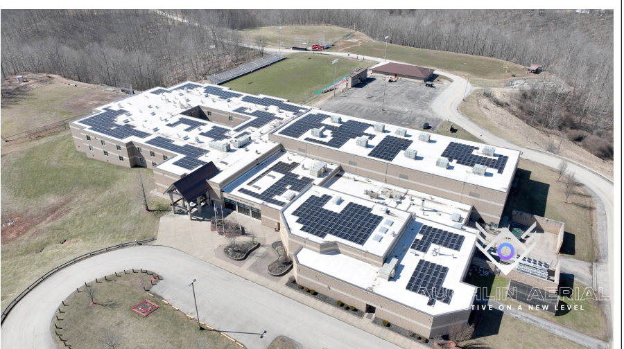
Courtesy Laughlin Aerial, LLC. Captured some photos of the recently completed solar project at Calhoun Middle/High School, a 596.6 kilowatt array was installed atop the building by Secure Solar Futures. A smaller 172 kilowatt system was installed atop Pleasant Hill Elementary. Calhoun County is the first school system in West Virginia to install solar on their school roofs.
