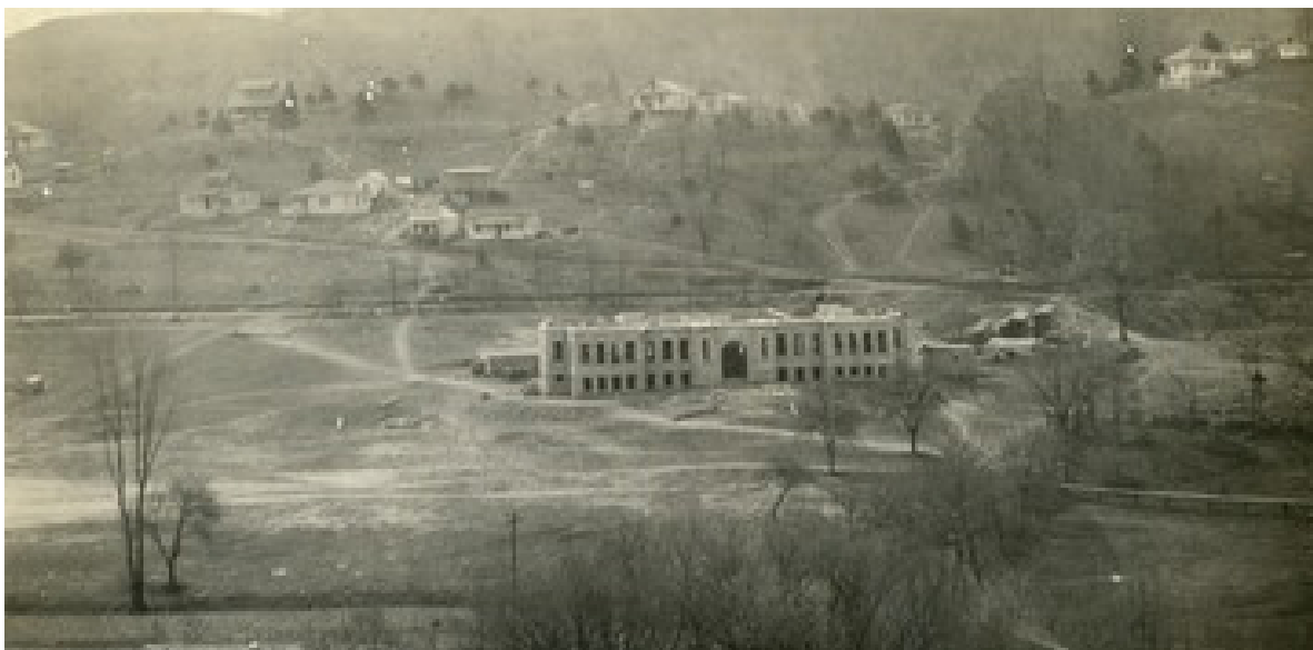
Calhoun County High School under construction in 1920. It opened to serve 70 children over a century ago. Next month the 1982 Foundation will celebrate work to revitalize the historic structure for a host of new purposes. Photo courtesy of WVU Online.
