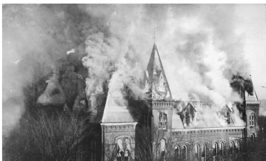
State building in Charleston was destroyed by fire.
