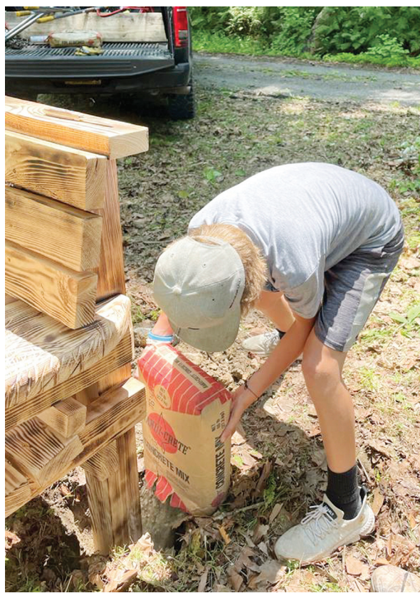
Tilyr gets the cement poured.
