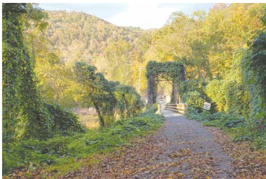
Trestle near Dundon trailhead.
