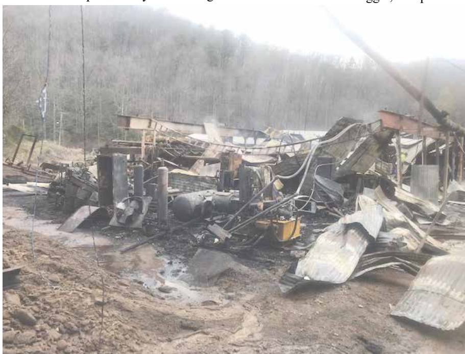
After the fire eleven months ago.
