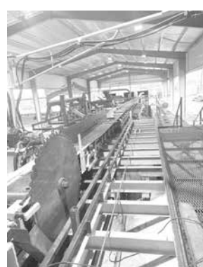
The new blade, lumber is first cut here.
