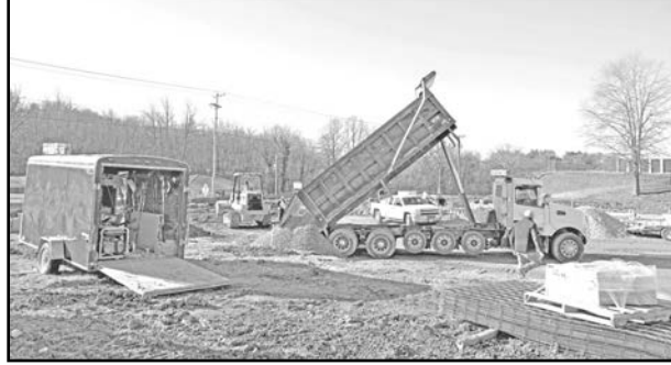
Taco Bell is building a new restaurant at East Vinton Plaza.
