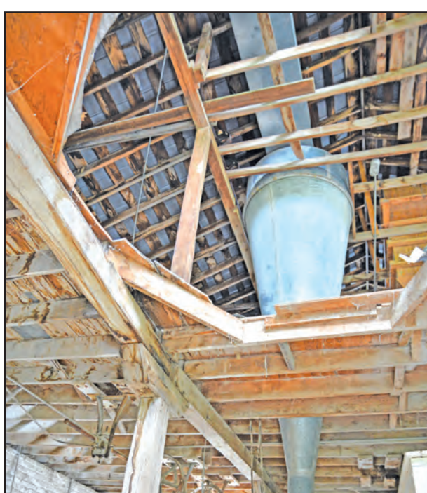
Milling equipment at the Gish Mill gristmill site
