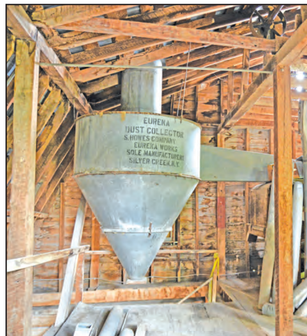
Gish Mill dust collector. Grain dust is highly combustible.
