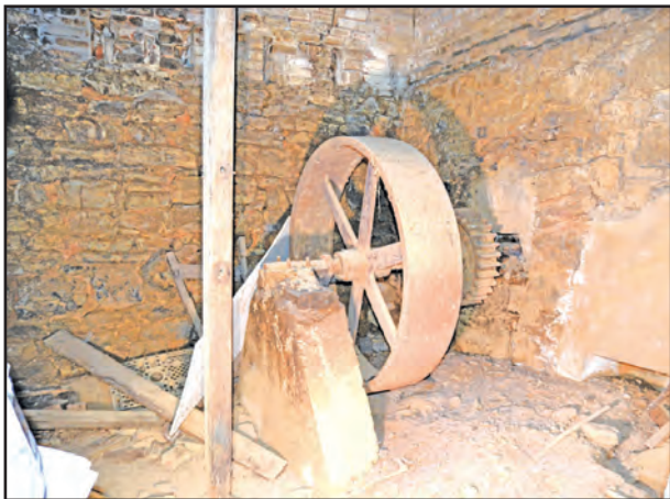
Gish Mill has been added onto several times across centuries and decades with the original structure dating from the 1850s.
