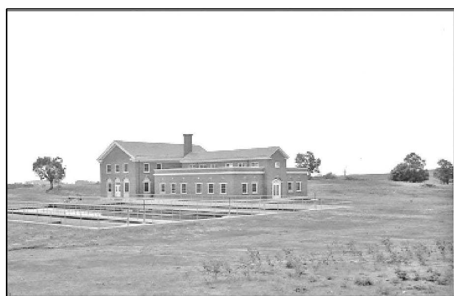
The Carvins Cove Water Treatment Plant first began operations in 1947.
