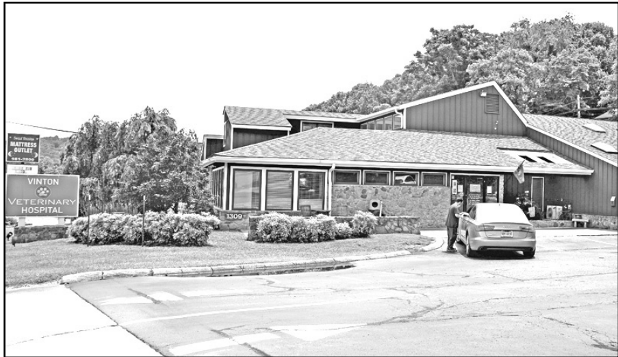
The Vinton Veterinary Hospital on Washington Avenue has announced plans for extensive expansion and renovations.
